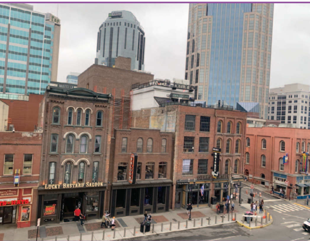
The brick-faced, turn-of-the-century row buildings that line the Lower Broadway strip now host many joints owned or licensed through big-name country stars.
