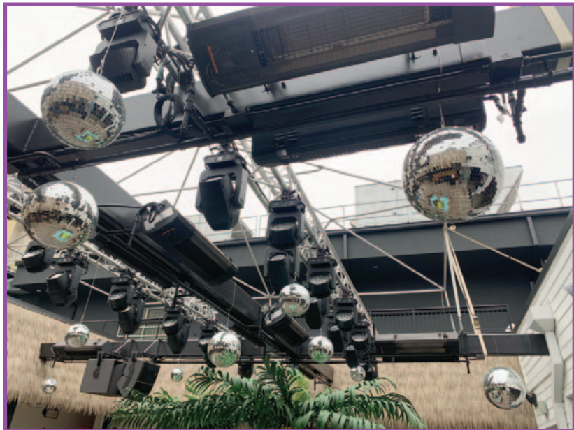
Gear on the roof includes, from CHAUVET Professional, eight COLORado 1 Quad Zooms, 25 Outcast 1L Beams, 23 Outcast R2X Washes, 12 STRIKE Array 2Cs, and four Color STRIKE Ms. Gear from ADJ includes six 15 HEX BAR IPs and eight 7P HEX units. Control is by a ChamSys MQ70.
