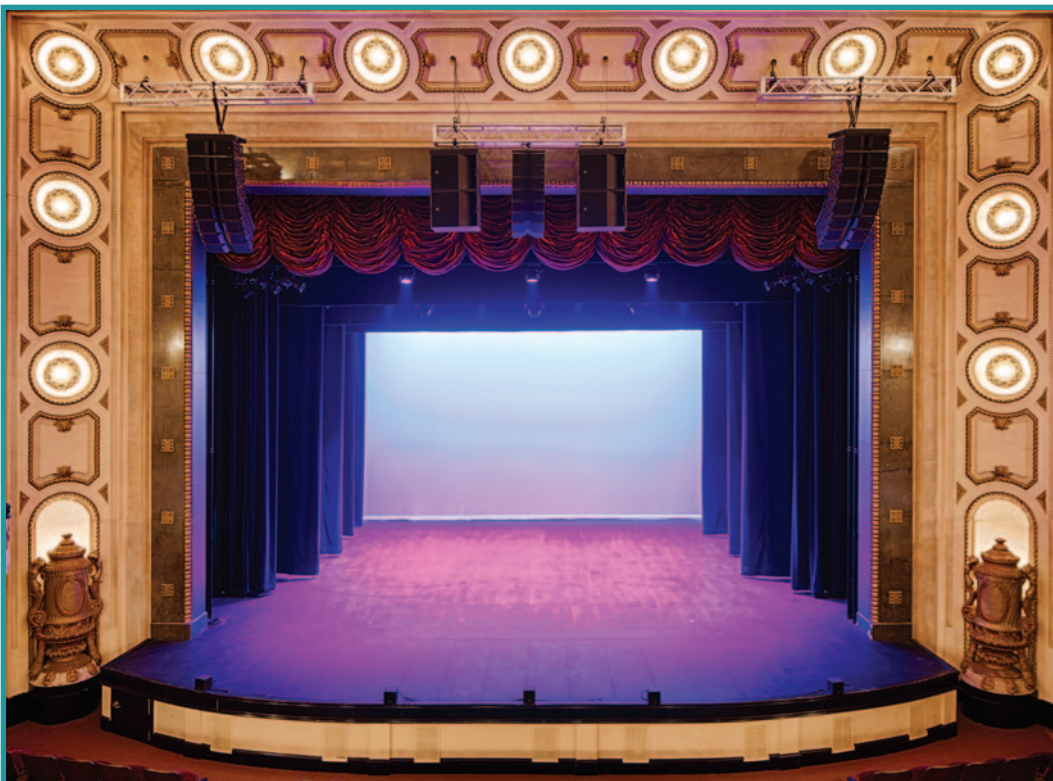
The automated rigging system comprises the proprietary Flyhouse Ease controls and winches developed and supplied by The Chicago Flyhouse, with variable-speed, cue-based operation; load cells; and slack line detection.
