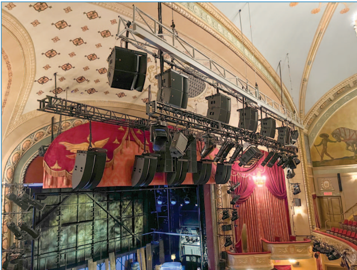
The frontal array of the musical's loudspeaker rig, for orchestra and front mezzanine seating, comprises five Scene hangs of L-Acoustics' new long-throw L2D arrays, spaced across the top of the proscenium.
